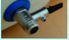
SMALL SLEEVE COUPLING: The tank is drained via the small sleeve coupling. Not only does this take a long time, it is also difficult to attach a hose to the sleeve coupling.
