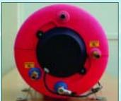
**USEFUL** labelling of the connection points on the tank. The insulation is unprotected.
